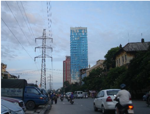
Hanoi – office bldg.
