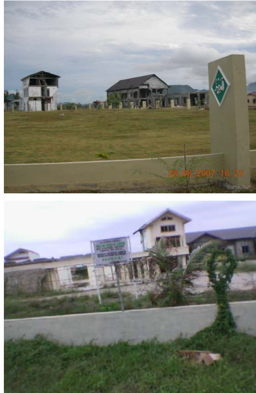
Figure 4. Destroyed buildings that are being kept intact as a memorial (as monuments). Top: buildings in a mass cemetery in Meuraxa, and above, the house that had been used to take amateur videos during the tsunami moment (Meuraxa).
