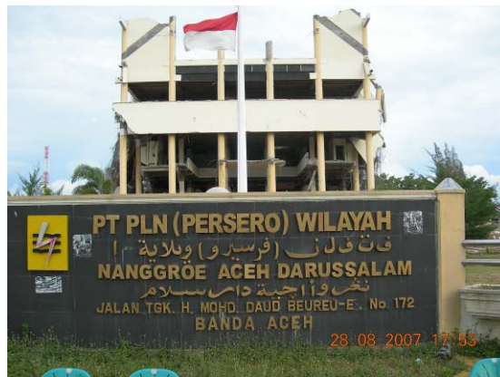
Figure 1. Remains of PLN Building under demolition (28 August 2007)
