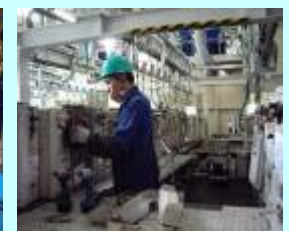
Recovery of refrigerant fluorocarbon from AC
